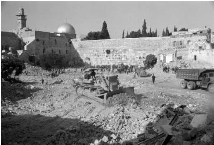
Figure 1. Demolition of the Mughrabi Quarter
